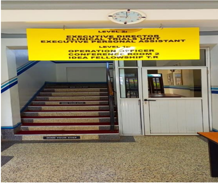
Figure 6: Stair case to Training and Conference Room
